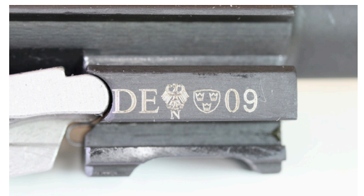
THE GERMAN PROOF MARKS ON A WALTHER P1 BARREL. THE THREE CROWNS INSIDE THE SHIELD REFERS TO THE COLOGNE PROOF HOUSE.
