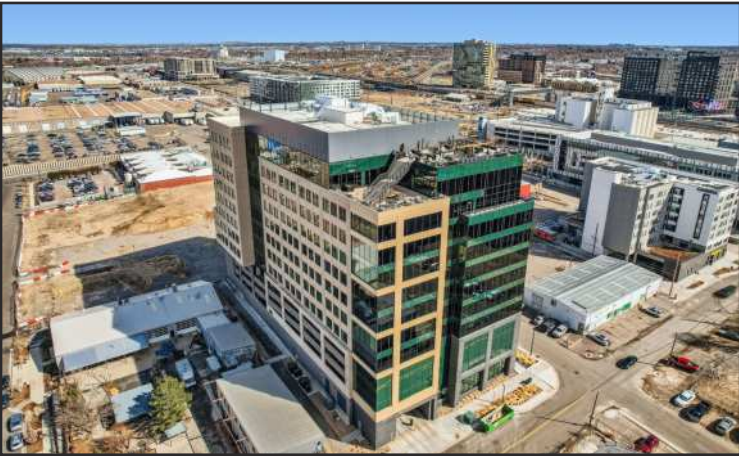
Developer and owner Schnitzer West has added new office and retail tenants at The Current, located at 3615 Delgany St., bringing the building to 63% leased.
