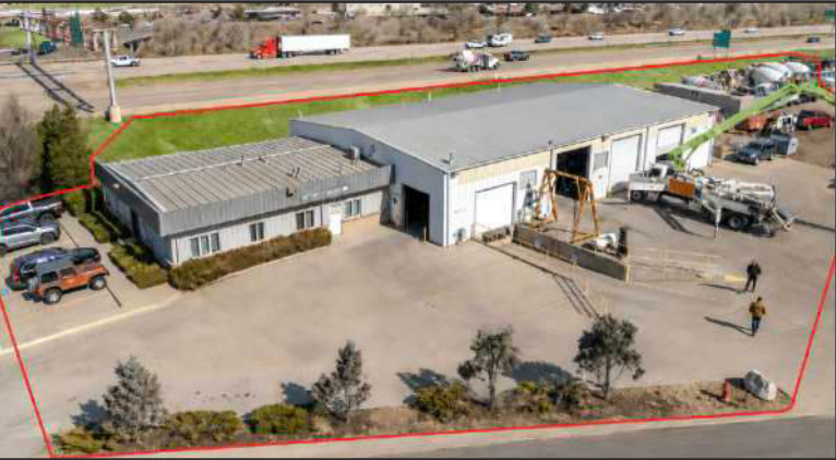
Jadian IOS purchased two industrial outdoor storage properties, located at 855 E. 68th Ave. in Denver (pictured) and in Mesa, Arizona, in a sale-leaseback transaction with Western Mixer in July.
