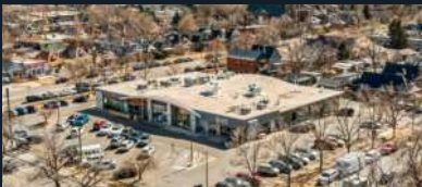
WASH PARK SUPPLY DENVER, CO
