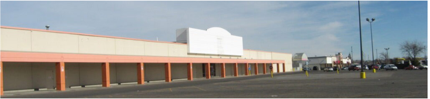
Developers of Caroline Ralston Creek pursued entitlement approvals to build 328 apartments on a former Kmart and Good Times site.
