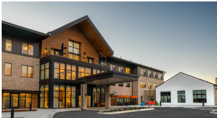
The Grand at Broomfield is an assisted living and memory support development, which the design team revisited a year after completion to determine if the building performed as intended.
