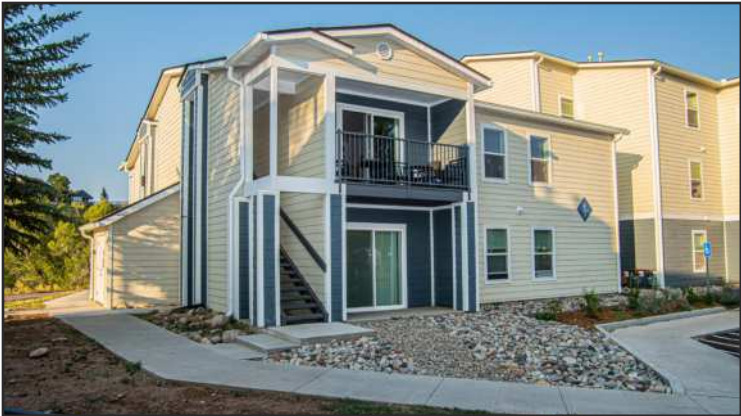
The 120-unit housing community serves families and individuals who earn 45%-60% of the area median income in Eagle.
