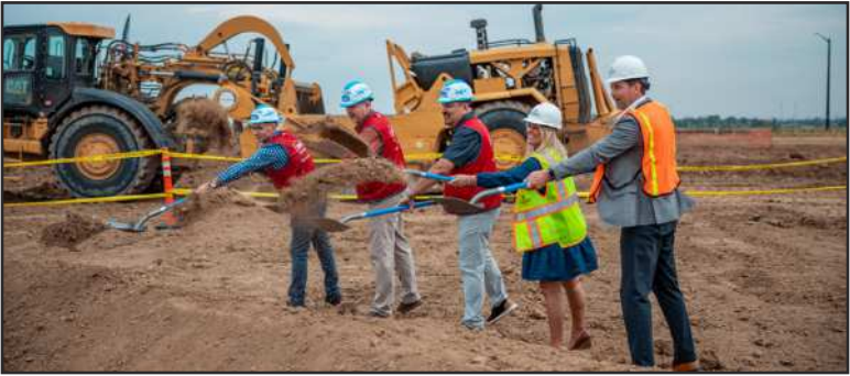
Lowe's staff members, Frederick Mayor Tracie Crites and Tyler Carlson of Evergreen Devco Inc. marked the ceremonial start of construction for a new Lowe's location at Silverstone Marketplace.
