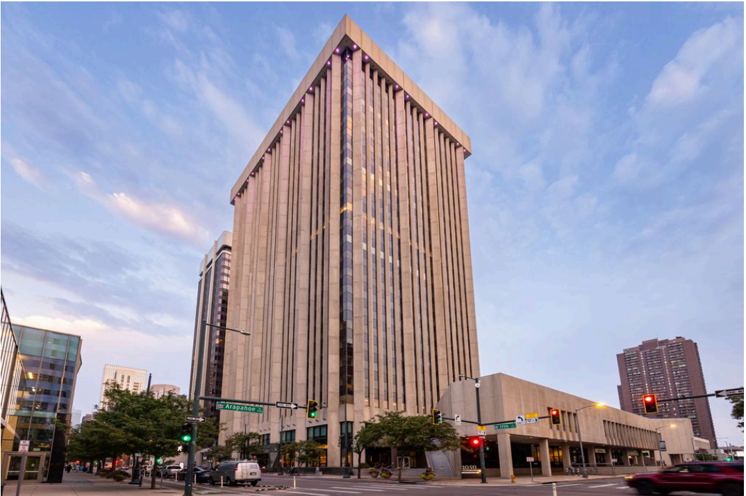
Paul Wedlake, University of Colorado Denver The University of Colorado, through the University of Colorado Foundation, acquired Independence Plaza from Independence Plaza Group Inc. for $27.95 million.
