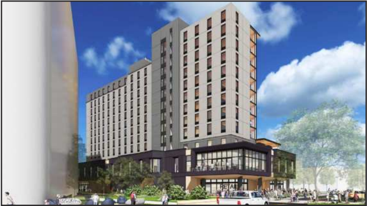
The 12-story, 150-foot-tall development features a two-story concrete podium supporting 10 floors of mass timber construction.
