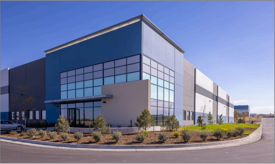
Opus broke ground on Sun Empire in Aurora in 2022.
