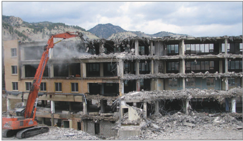
Boulder Hospital decommission
