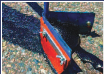
CRACKSEALING
