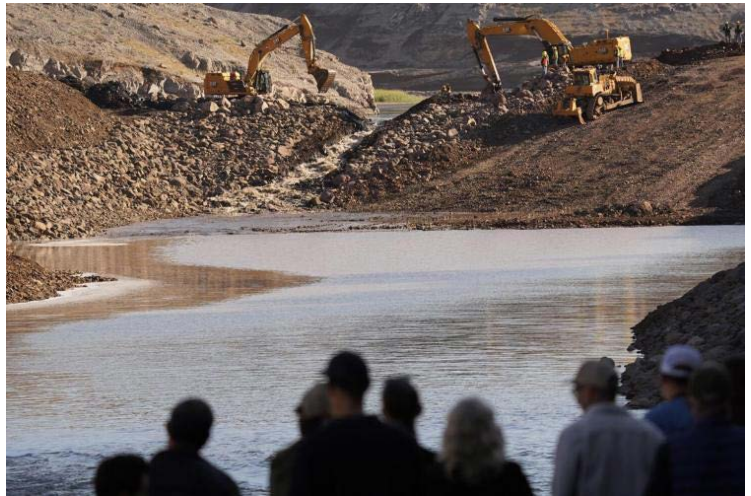
(Left) The removal of four large dams from the Klamath River allows salmon to again reach about 400 miles of their original habitat that had been blocked for many decades. Photo: Jason Hartwick/Swiftwater Films. (Right) Heavy machinery scoops away a cofferdam that diverted Klamath river water while crews worked on the first of the four Klamath dams that have now been removed. Photo: Matt Maise/Yurok Tribe.
