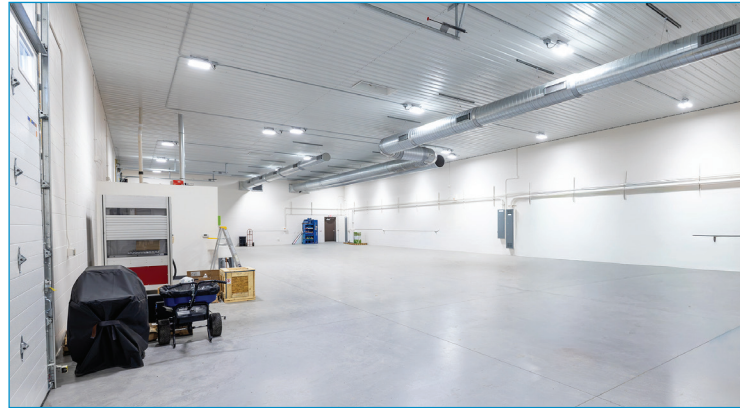
The recent 6,000-square-foot addition brings Sheridan's total facility to 10,000 square feet. The space is held at a constant 72°F year-round, supported by an oversized HVAC system that stabilizes ambient temperature for precision tooling work.
