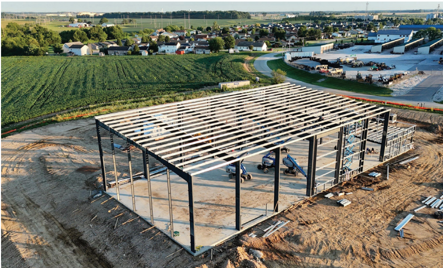
Construction began on Haidlmair's newest facility, which will be located in Greensburg, Indiana, earlier this summer.
