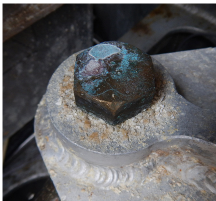
Galvanic action between metals. Page 30.
