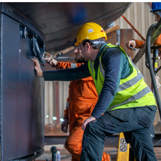
The keel of the Oceanus 12 is largely for holding the skin cooling tanks for the boat’s generators.
