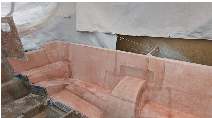
The added buoyancy and unique shape of the new after section were clearly visible before the deck and internal structure were installed.
