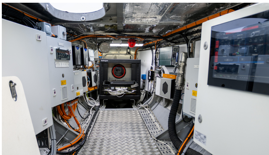
Facing Page —The latest Oceanus 12 in Plymouth. Left —The interior reveals accommodations for the 350 cables that snake through the hull connecting generators, batteries, sensors, communications components, computers, and actuators, but no crew.
