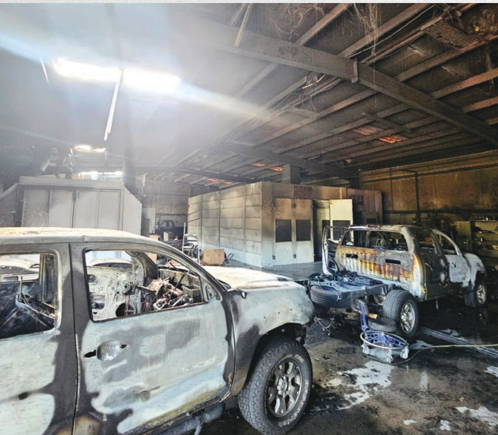
Above: 1981 news article reporting the fire at the original Stan's. Below: Destruction to the body shop as the result of the 2025 fire.
