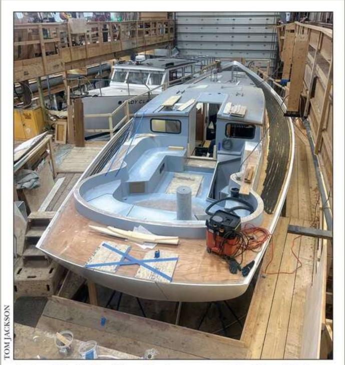
At Brooklin (Maine) Boat Yard, a custom 56' cold-molded cruising yacht is on track for launching in June, only eight months after her hull molds were set up in September.
