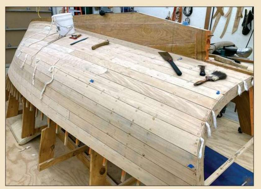
7. Once the planking was completed, it was time to fair and sand the hull. One advantage of planking the hull upside down was that, as tedious as fairing is, it is easier to do working down. It is also easier to see the hull's surface with direct light. After chalking high and low spots along individual planks, Sandy used a scrub plane to shave high spots and then smoothed the surface with a sanding long-board, continuing with both tools judiciously until the hull was smooth and fair.
